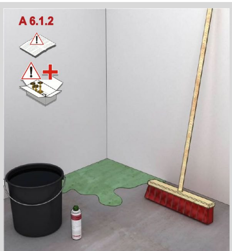
Picture 5 Application of the subfloor sealant
